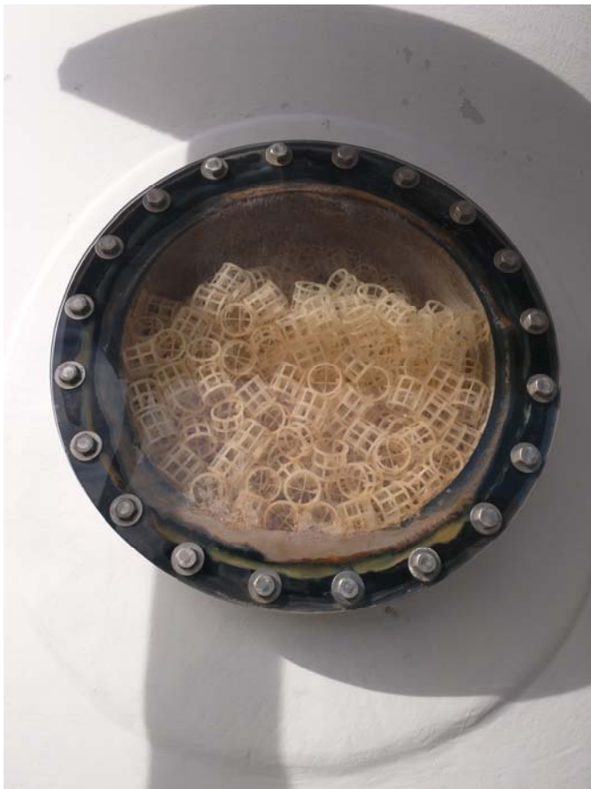
Figure 36- Area 12 tower view port, showing packing material
