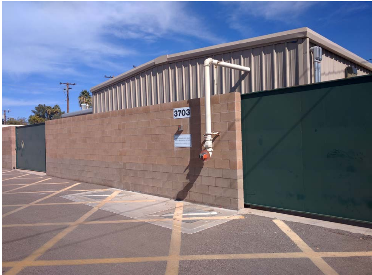
Figure 17-Area 7 Treatment Facility exterior
