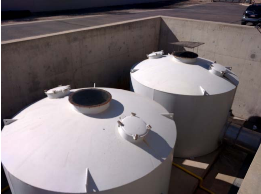
Figure 15-MRTF carbon adsorption units
