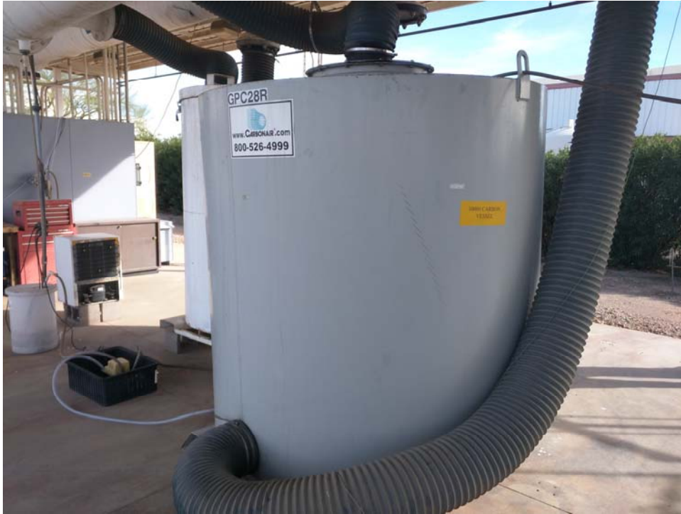
Figure 35-Area 12 Carbon adsorption vessel
