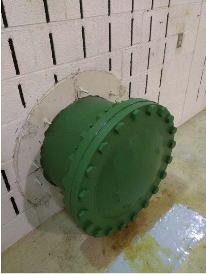
Figure 13-Former connection to well PCX-1, now capped off
